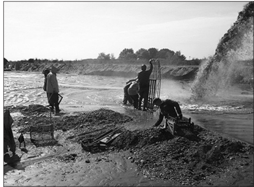
Figure 2 The outcrop in Langenboom (municipality of Mill) is an underwater sandpit called 'de Kuilen'; sand is dredged from a depth up to maximum 20 meters, using a stationary suction dredger; pumped ashore through a floating pressure pipeline and dumped into large sand depots adjacent to the lake. [photo: Rene van Vliet]
